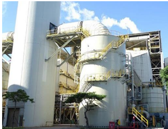
Power Plant of Nanya Plastic Corporation
