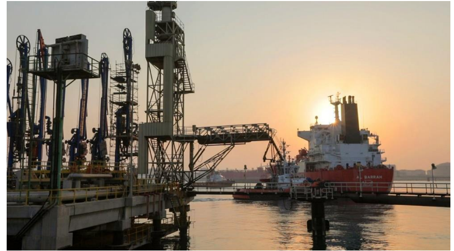
Blue Ammonia Carrier at Jubail terminal in Saudi Arabia
