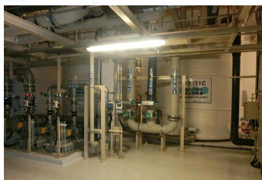
▲ DIR Drain Reclaim To UPW system
