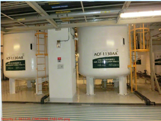
▲ Acid waste drain water reclaim to RCW
