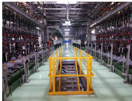
EDR Water Recycling Pipeline Project
