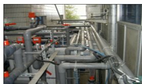
Recovery of cooling water from electronics manufacturing factory by EDR process (Tiger company) (550 m 3 /day)
