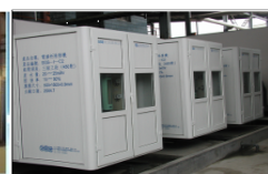
EDR desalination of high conductivity river water for process water ( 2400 m 3 /day)
