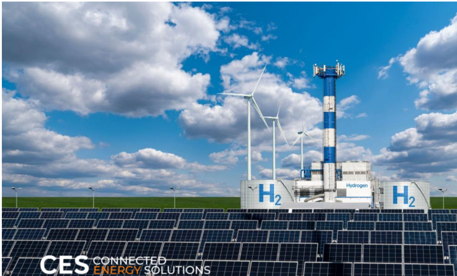
New green hydrogen generation plant commissioned in Germany September 16, 2022
